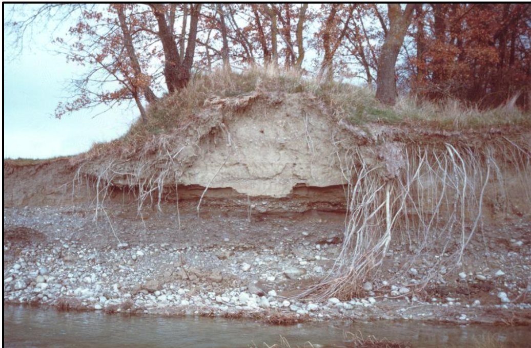
Figure 1.3: Cantilever blocks reinforced by roots in Cecina River Italy (Papanicolaou et al., 2006)
